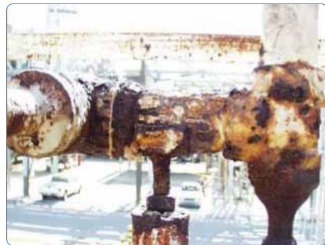
Industrial environments will promote significant corrosion of carbon steel piping components
