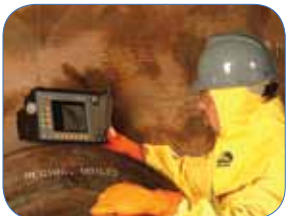
Phased array ultrasonic testing of reactor vessel and piping systems.
