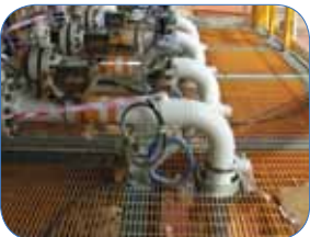
Rightrax™ installed-sensor system continuously monitors wall loss due to sand erosion at critical elbows on production platforms.
