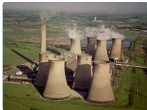
Remote Visual Inspection provides recordable, indexed, high quality documentation
