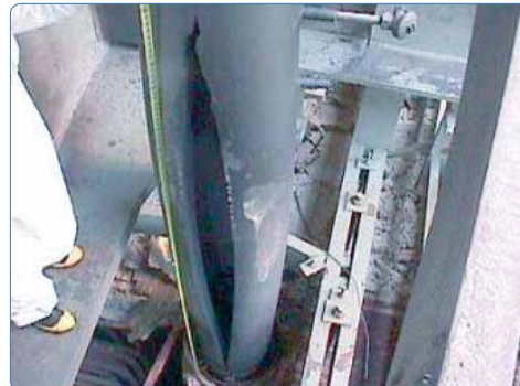
Elevated temperature damage can occur with increasing age and operation severity
